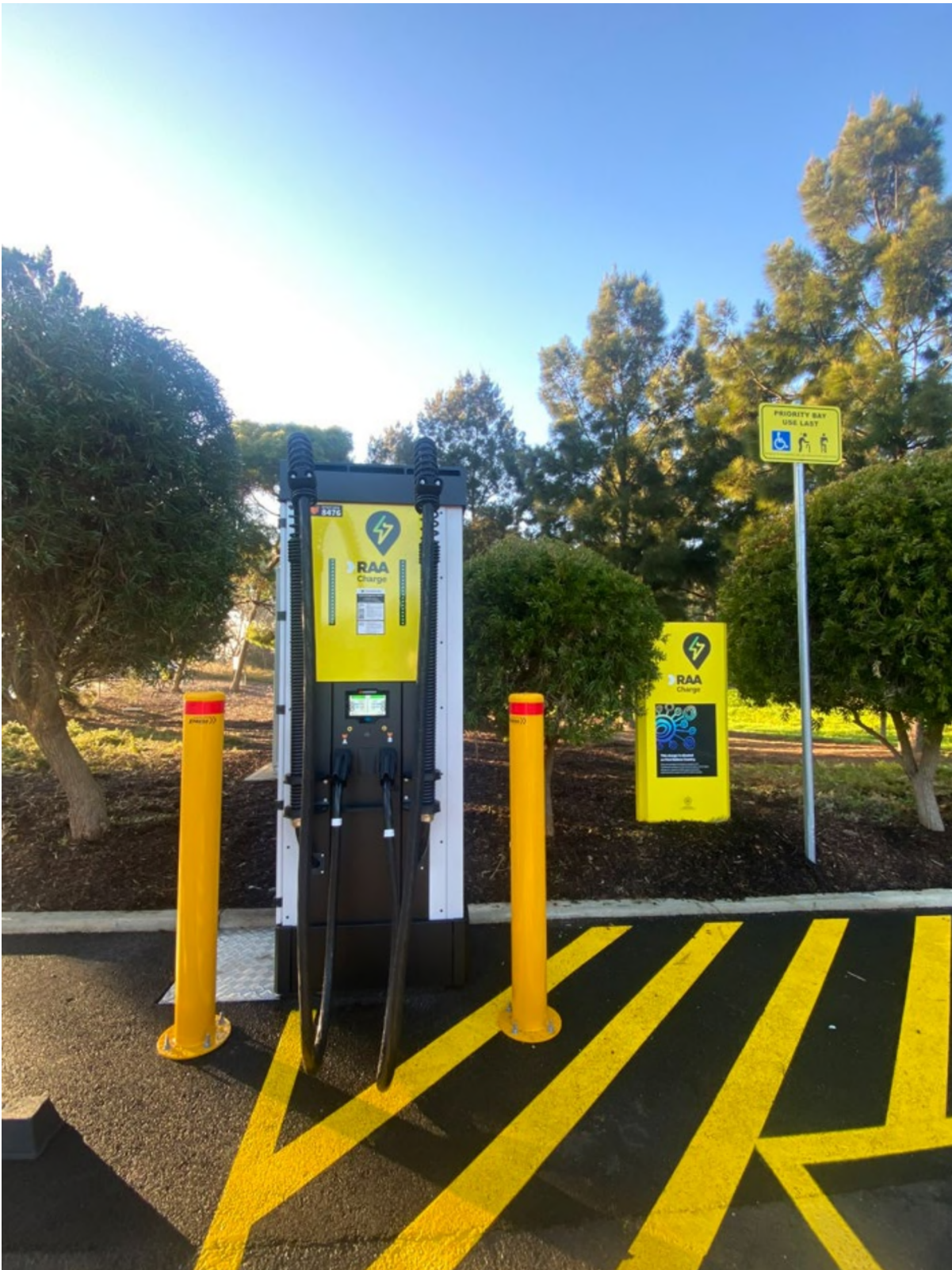
Kempower Rapid DC charging unit with two plugs.
