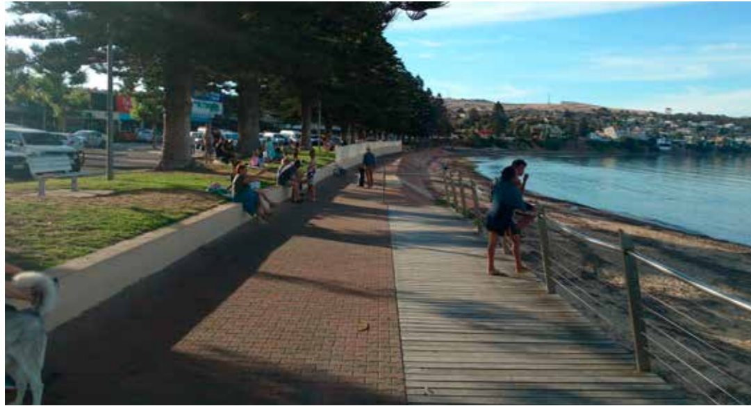
The Parnkalla Trail runs the length of the foreshore with retaining walls varying in size + materiality providing informal seating opportunities.
