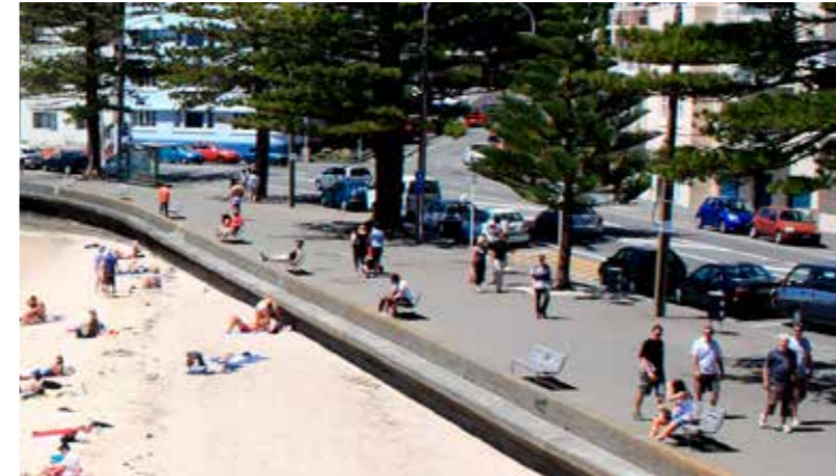
A new sectional, pre-cast sea wall panel is to be designed for the central portion of the foreshore to enable deflection of wave action and provide informal seating.
