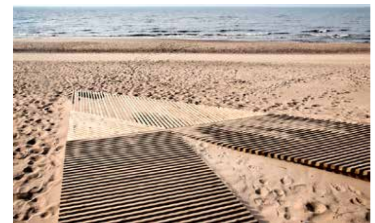
Timber slat surfacing of sand for access through revegetation and for DDA compliance.
