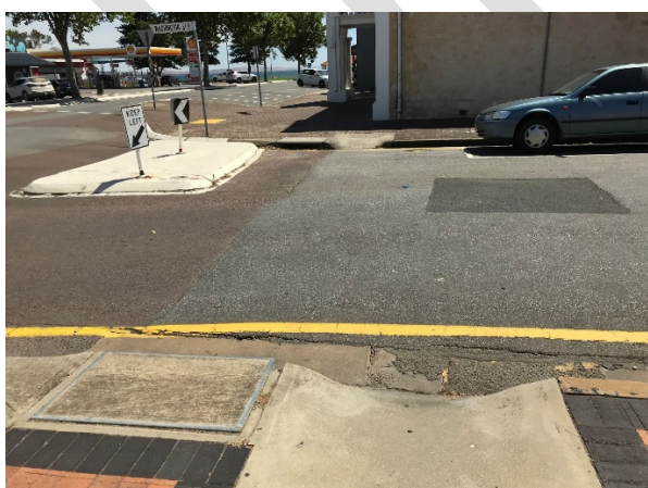
Photo 5: Kerb ramps difficult for wheeled mobility device and do not line up Photo 6: Parnkalla Trail blocked off
