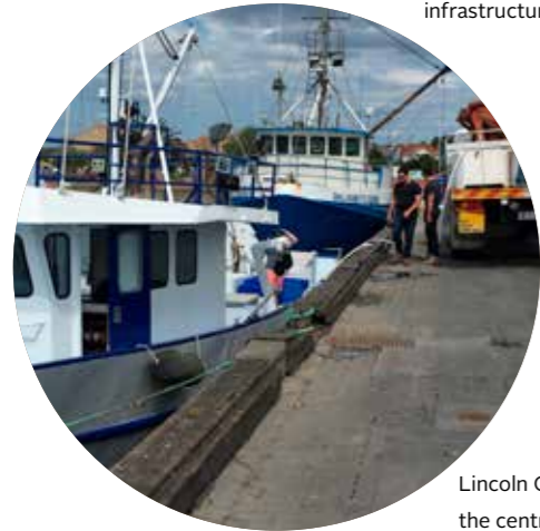
Some CBD streets and public spaces have ageing infrastructure.
