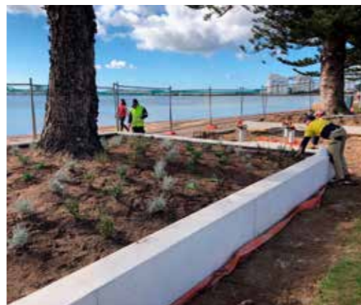
Local contractors installing planting to raised planter bed.
