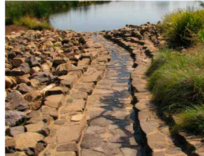
Formed rock spillway using locally sourced material.
