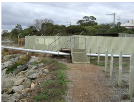
Steep ramp over oil pipeline
