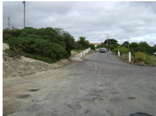
Existing ramp section
